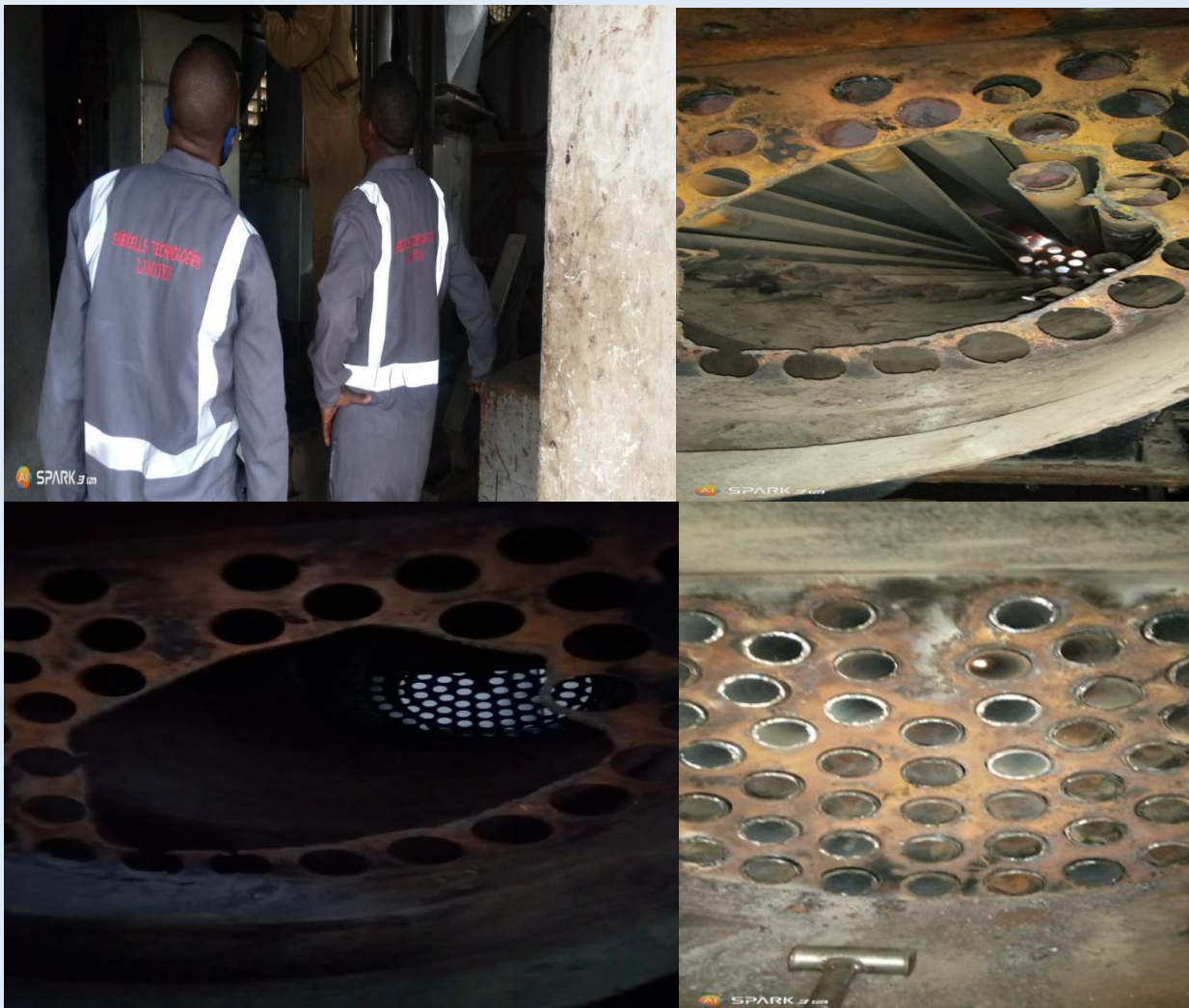
Boiler APH Re-tubing at coastal bottlers ltd (coca cola) in mtwapa
