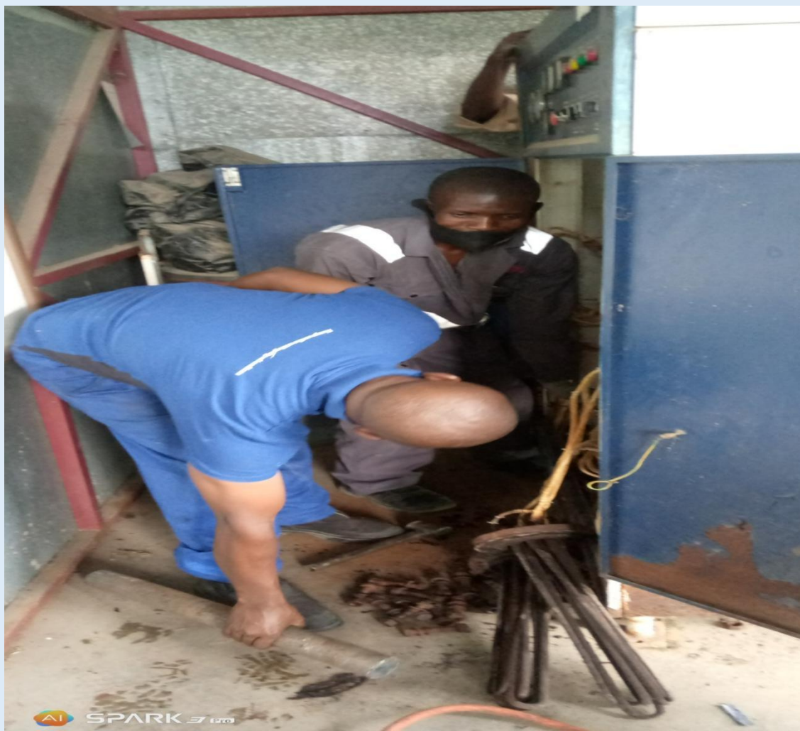
Boiler service work at flamingo Horticulture in Naivasha
