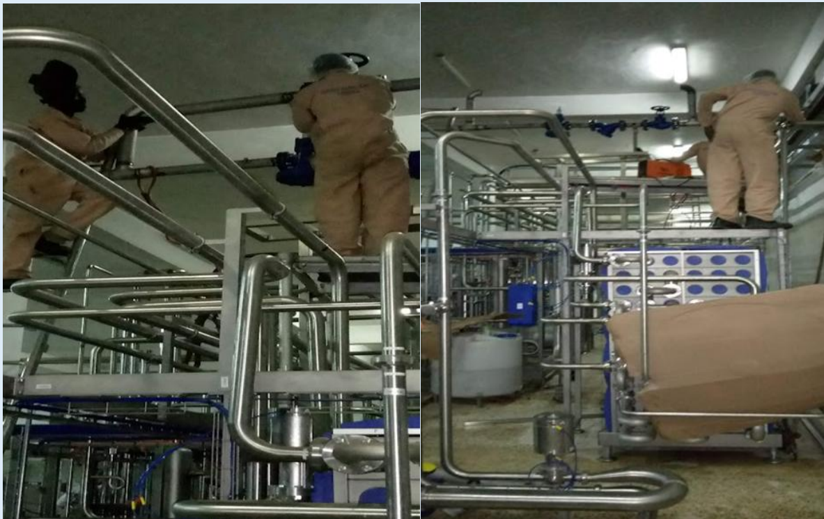
Piping works (milk plant)
