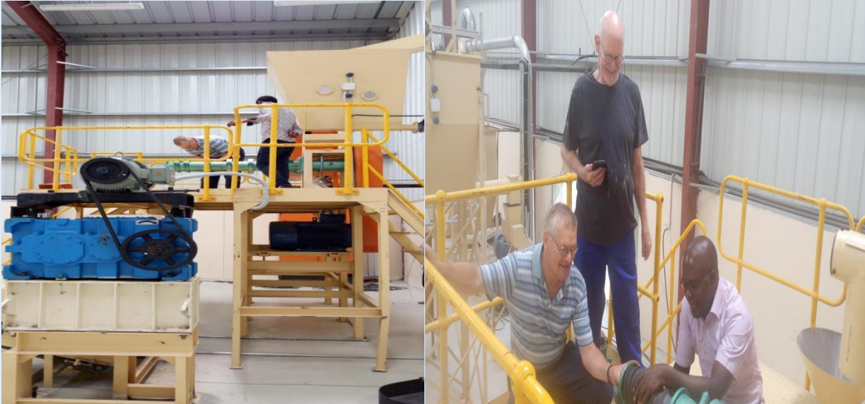
Soya milling, extrusion and oil pressing plant installation in addis ababa
