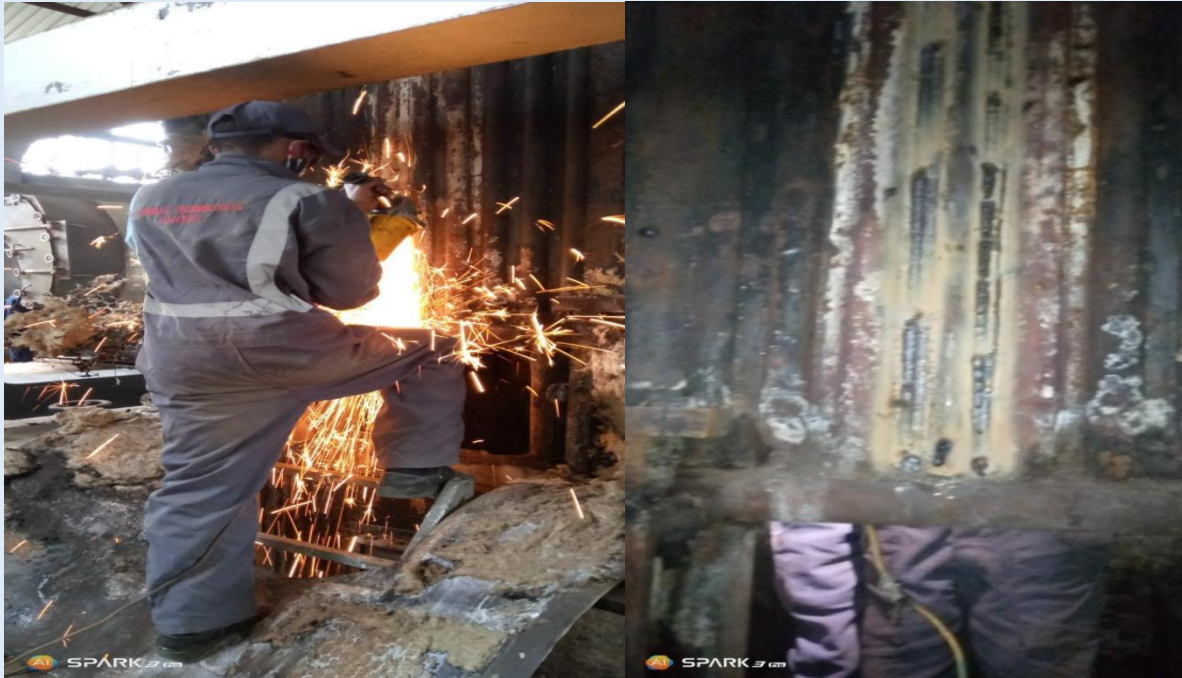
Boiler repair and re-tubing @ Uplands dairies
