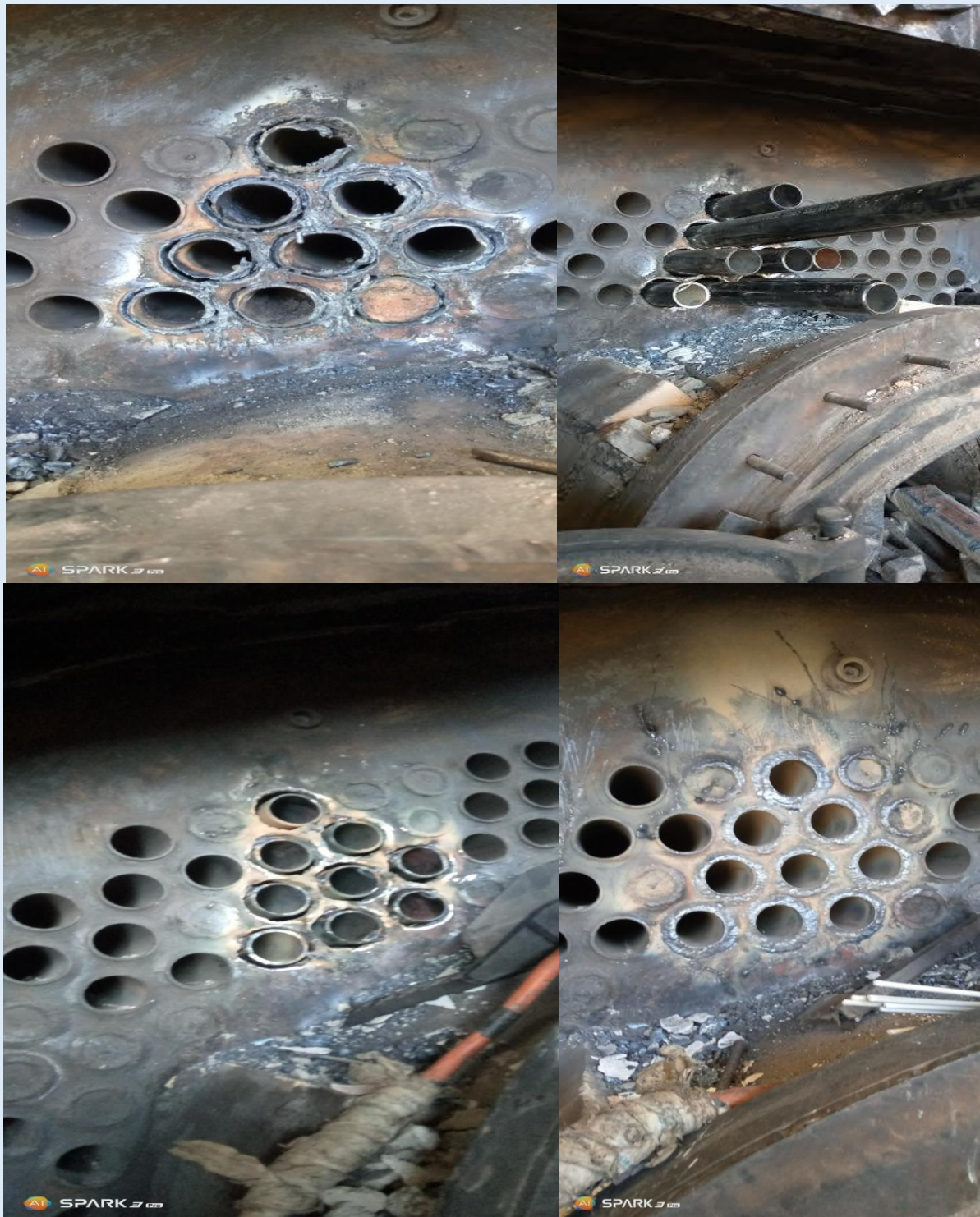
Boiler re-tubing at spinners $ spinners ltd in Ruiru
